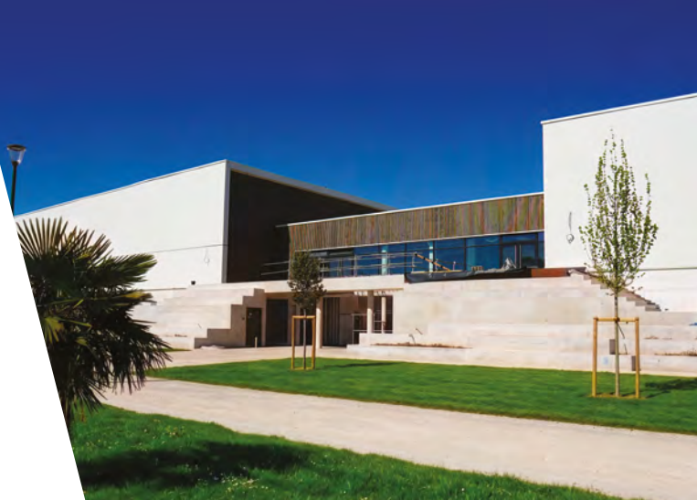
Restructuration du gymnase Jean-Bouvin
